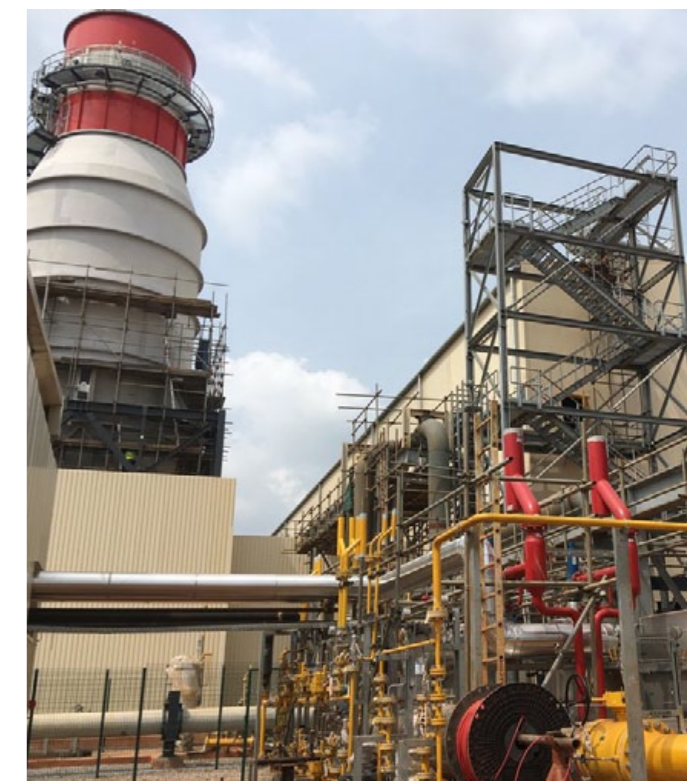
Azura Power Project - Benin City, Nigeria
