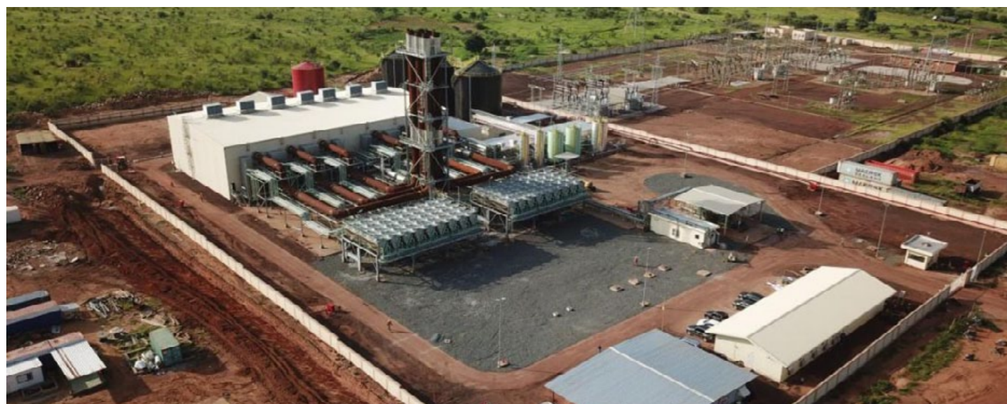
90 MW Thermal Power Plant in Kayes, Mali
