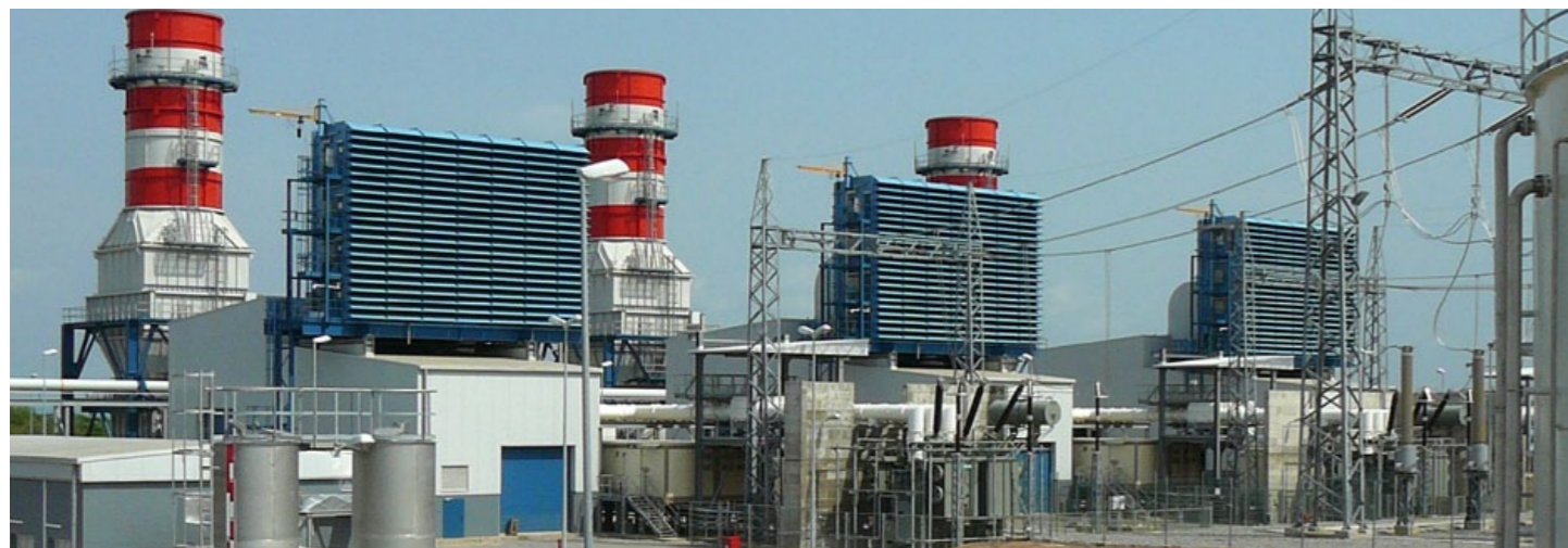
Azura Power Project - Benin City, Nigeria
